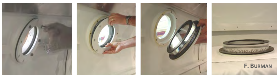
Removing chamber windows for inspection
